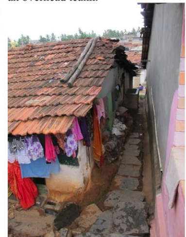
d) No apparent use. No visible signs of water near or outside house.
